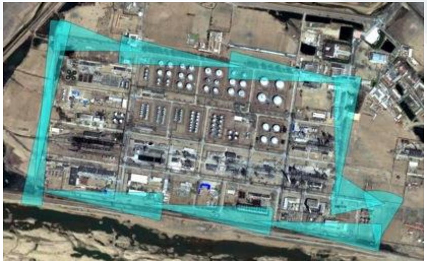
Simulation of camera setup. This is not a real installation.
